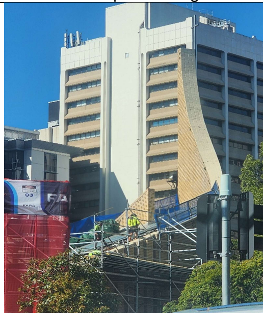
Ongoing roof construction work
